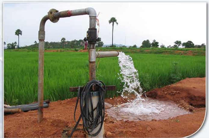
International Development Enterprises (India) demonstrated a project to promote micro-irrigation technologies that helped reduce energy consumption in the range of 15-30% by using energy-efficient sprinklers. The project was supported under USAID's earlier Small Grants Program (2004)
