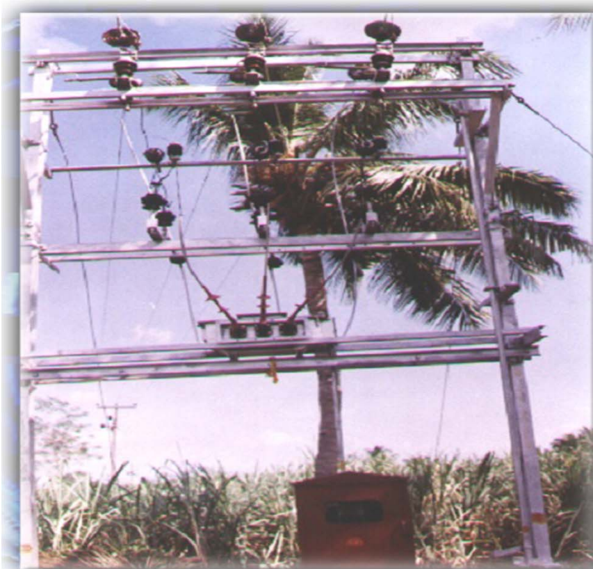
Original 3ph 100KVA Dist. Transformer replaced with 11KV. CTPT set
