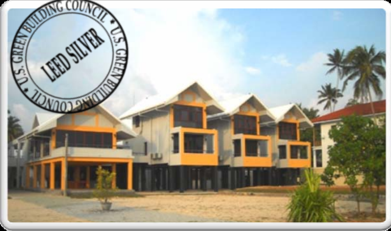
VTA SCHOOL, AHANGAMA
