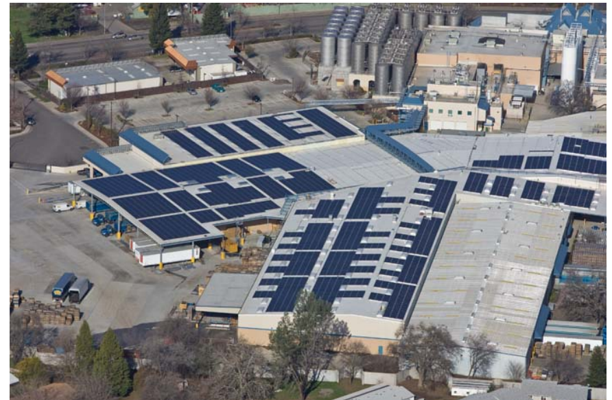
Photo: Brian Peterson, Sierra Nevada Brewing Company, Chico, CA California Solar Initiative Funded System, 1,258 kW, September 2007 Installer: Chico Electric
