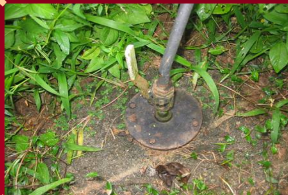
Biogas plant (gas outlet)
