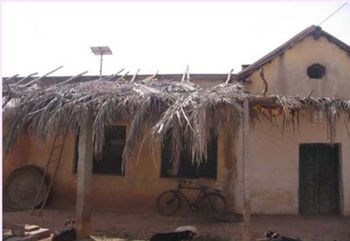
Solar PV panels on silk rearing centres
