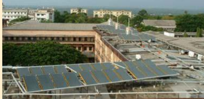
Right: MAHE - Hostel Solar Water heater installation; largest water heater installation in the country
