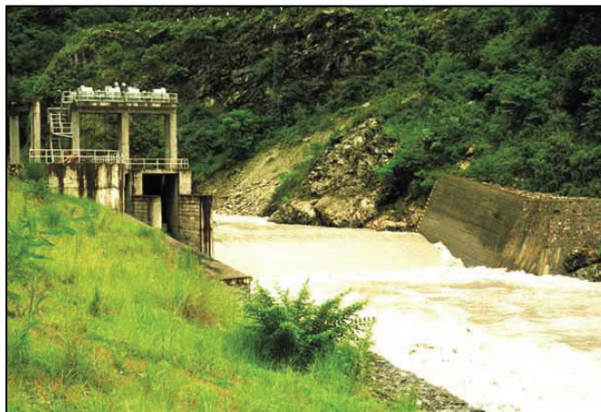
Typical Small Hydropower Installation - Nepal
